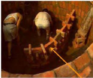
**Figure 3:** Internal baffle wall (KfW, 2009)
