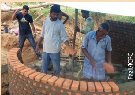
An open dug well under construction in Kiran, Batticaloa south. 2013
