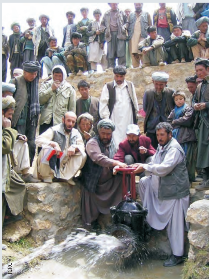
Opening the valve of the dam built by ICRC in Shaidan village, Bamyan province
