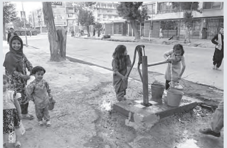
Hand pump installed by ICRC, Kabul city 1994.
