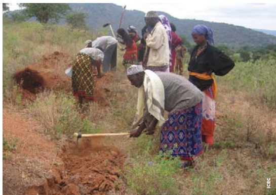
Community members in Moyale dig trenches which are then filled to prevent soil erosion during the cash for work project
