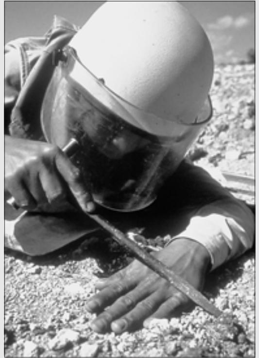
Cambodia 1995, Detection of buried mines usually requires probing every few centimeters of soil over vast areas of land © Handicap International
