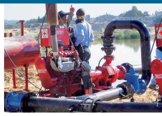
Emergency pumping system being set up in Beit Lahia to prevent the banks of a wastewater reservoir from bursting
