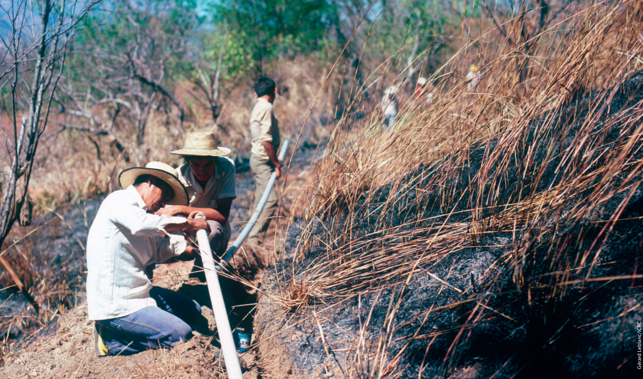
Pipes being laid to supply villages with clean water (left).
