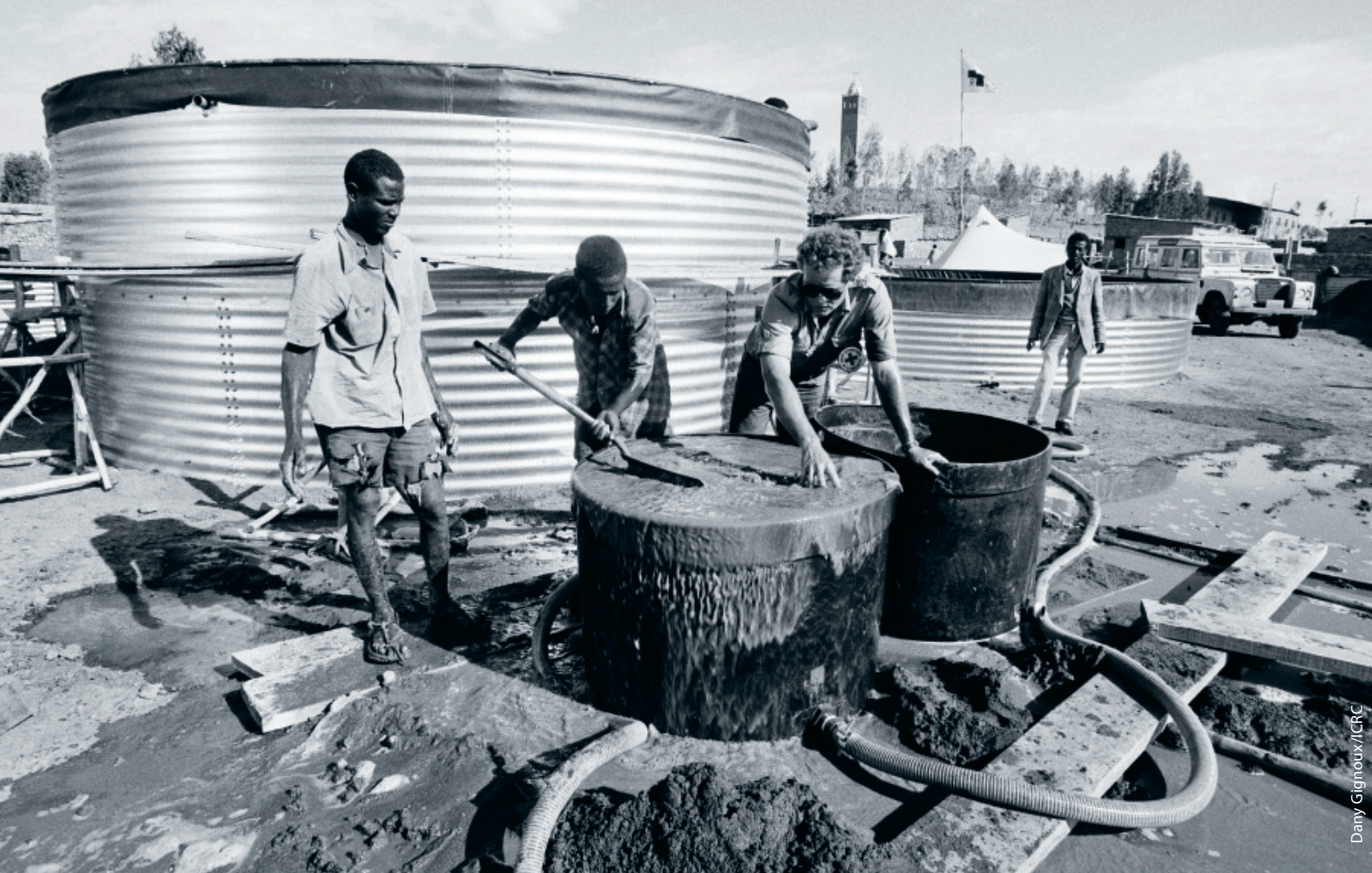
Tigray, Mekele. Installation of a sand filter next to a water reservoir.
