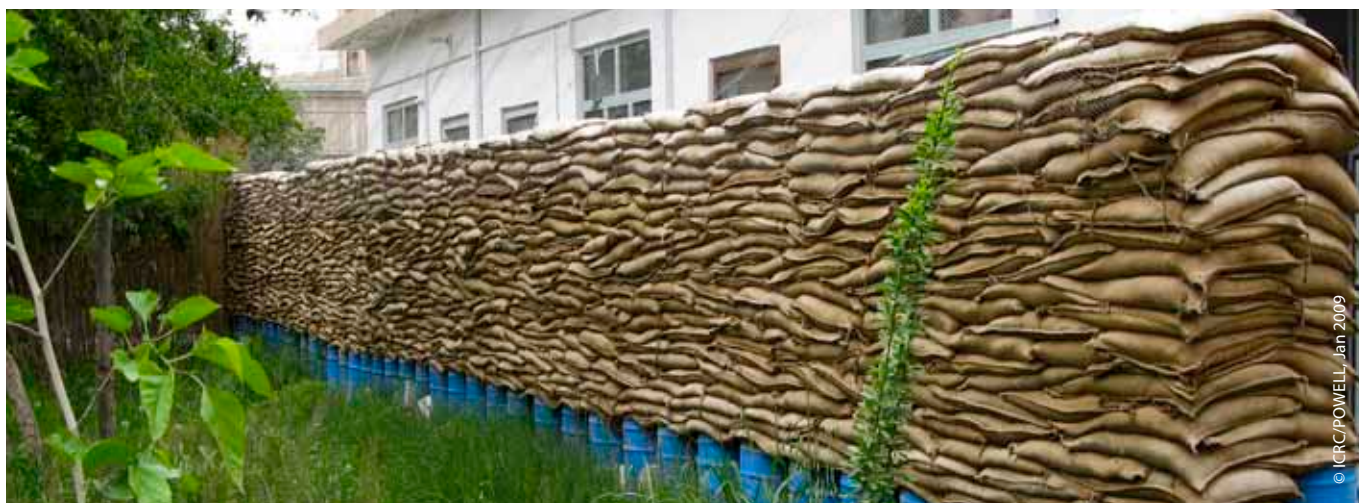
Afghanistan, Kandahar: Sand bags protect the entrance to an ICRC building from possible blast damage.
