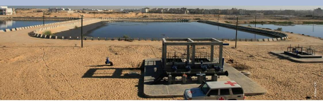
For several years, the Rafah wastewater treatment plant has been insufficient for treating the sewage of the city because it was too small, too old and needed repairing. The sewage network covered only part of the city and the effluent discharged to the sea was almost untreated and without the possibility of reuse.
