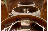
**Figure 2**: 100 m<sup>3</sup> digesters in series (Rwanda; Mottet, 2009)
