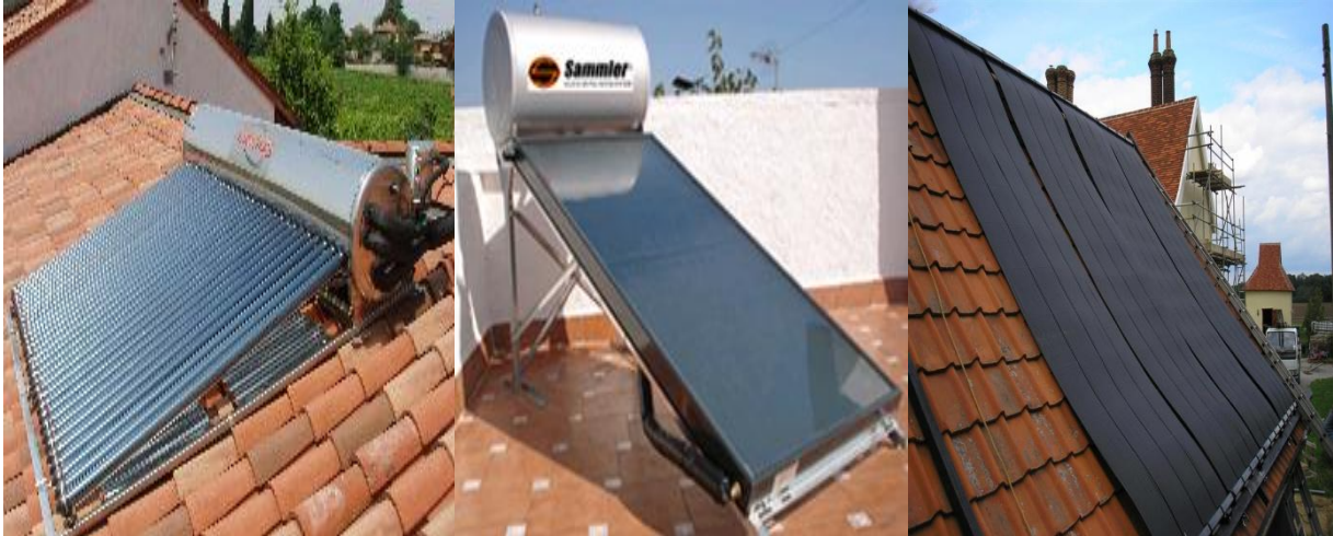
Figure 7: Vacuum tubes collector
