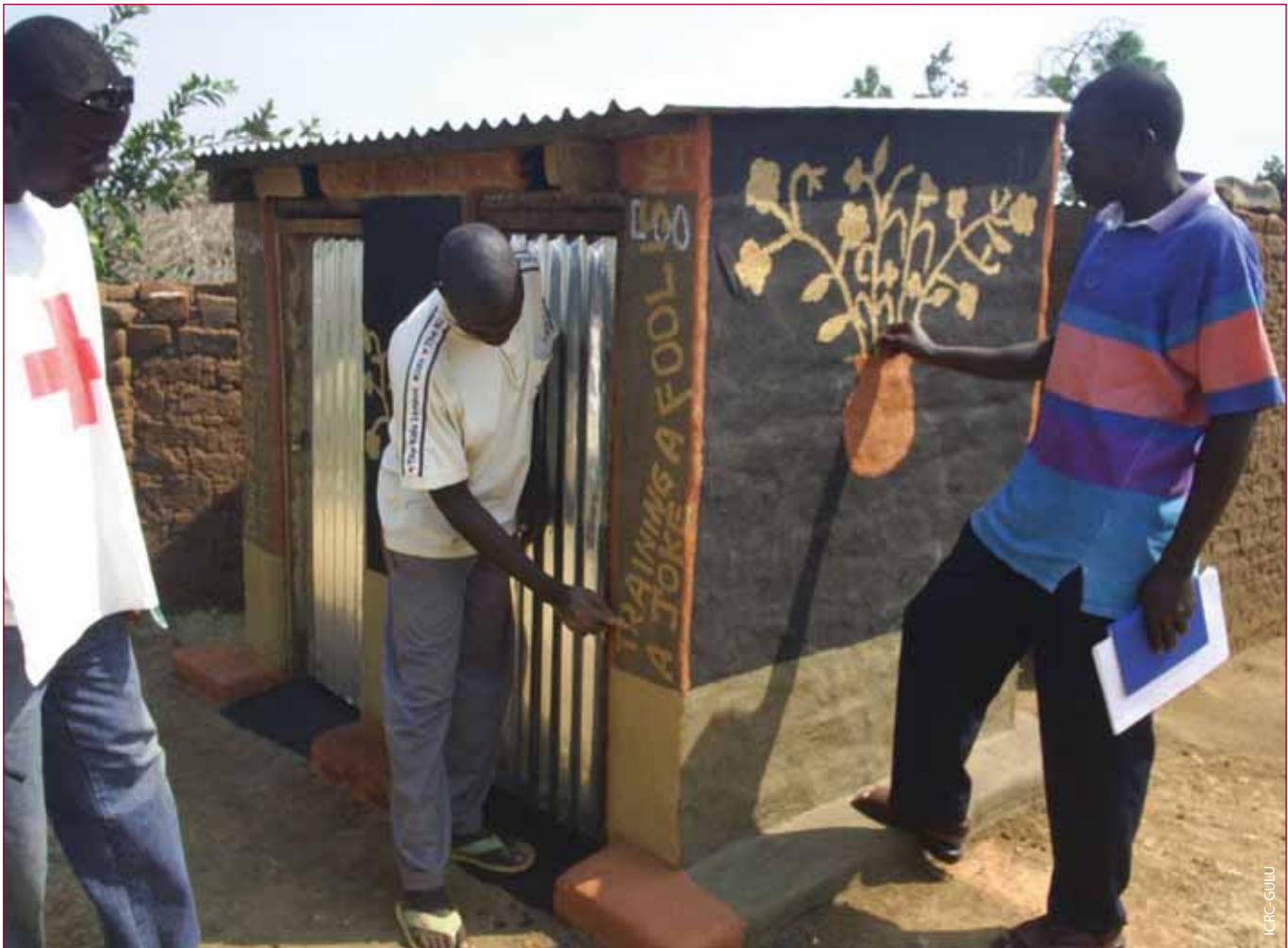
Latrine construction at Pabbo camp in Amuru District
