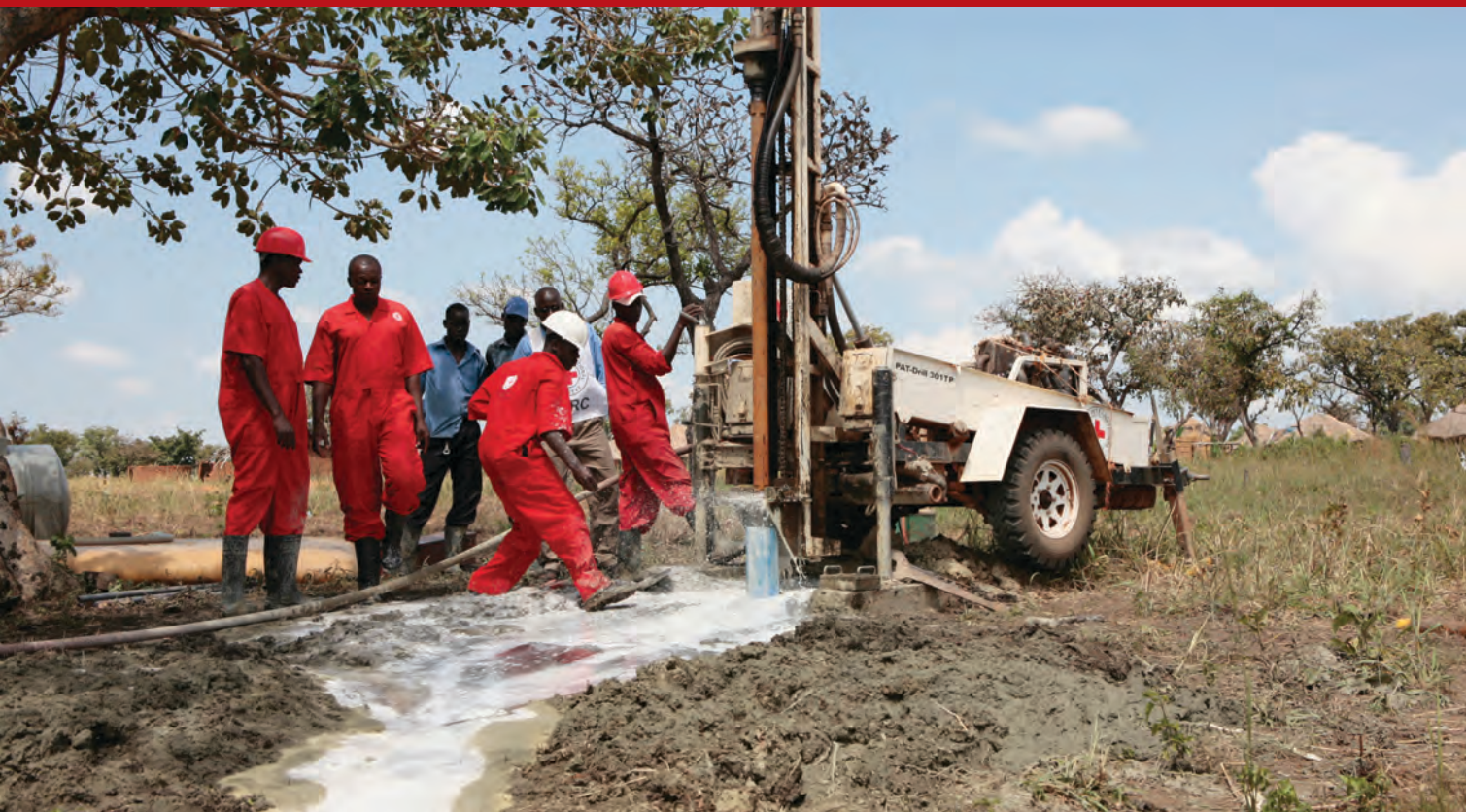
ICRC staff drilling a borehole at Laminajiko in Pader District
