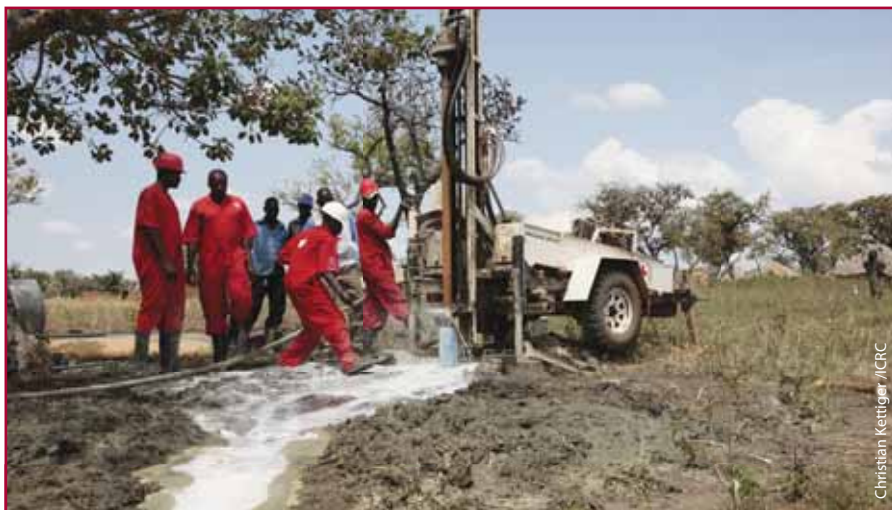
ICRC staff drilling a borehole at Laminajiko camp in Pader district
