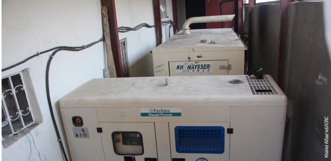
Two generators were delivered by the ICRC to al-Mudhafar Hospital in Taiz, one 150 kVA generator and one 60 kVA generator as emergency support after the two existing ones were totally destroyed.
