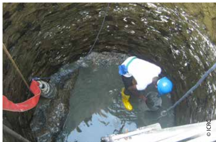
Well cleaning in progress.
