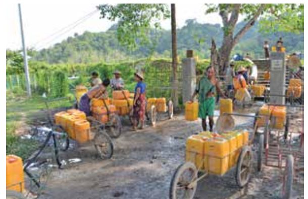
ICRC's rehabilitation work of water sources benefited the local communities.
