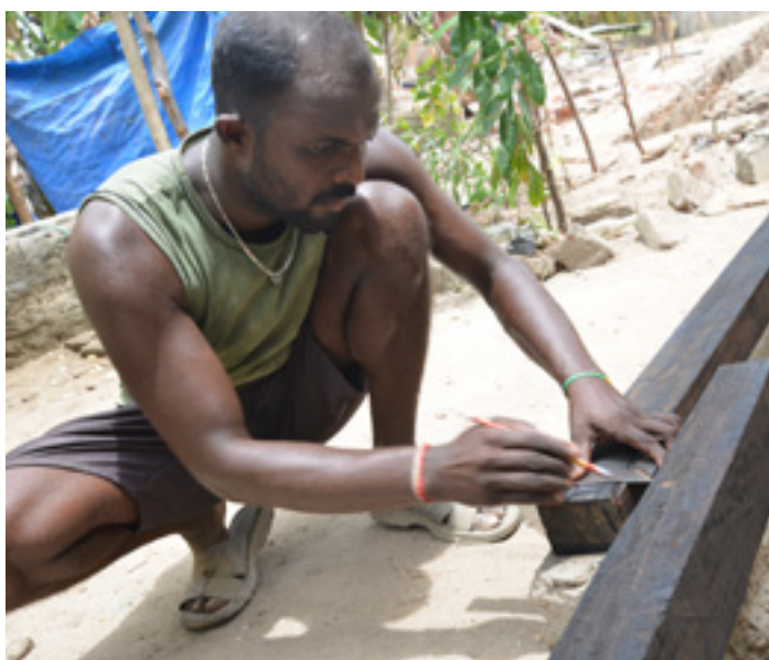
Chithravel constructing the roof of a house.
