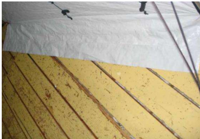
Picture 11- Sleeve sections for the sloped pipes
