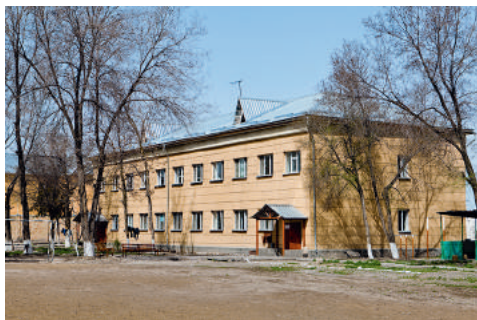
Renovated buildings for patients with non-contagious form of tuberculosis in Penal Institution-31
