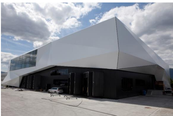
The Logistics division at Headquarters, Satigny (Switzerland),
