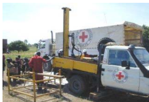
The ICRC drilling a borehole at Kitgum
