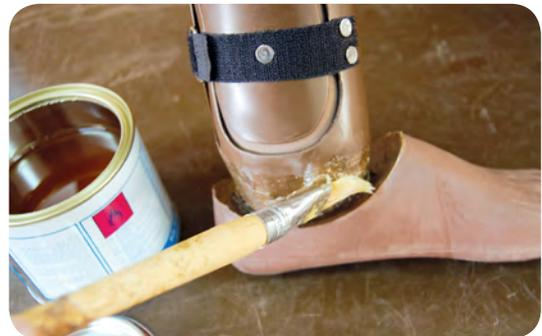
Fill the gap between the socket and the foot with EVA
