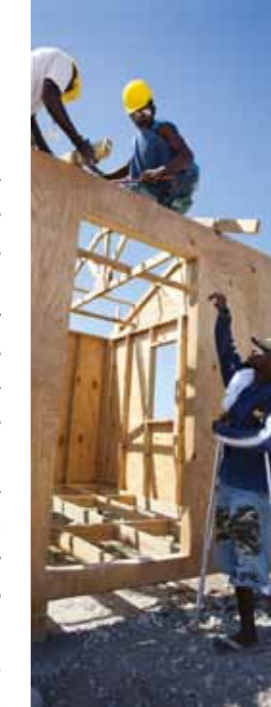
☞ At the La Piste camp in Port-au-Prince, the IFRC supported a team of builders, all of whom are deaf, to construct shelters in 2010. Photo: Ben Depp/IFRC
