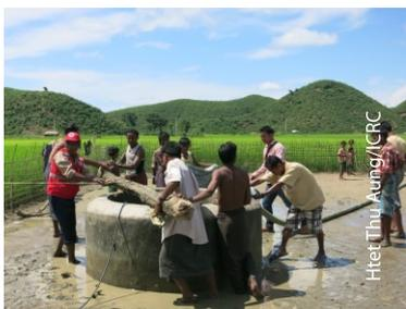
**A well from Pu Rein village in Mrauk-U township being cleaned with the help of an ICRC sludge pump.**
