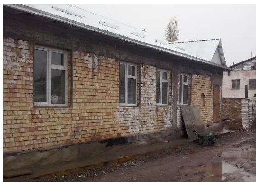
Construction works in SIZO 53, Jalal-Abad
