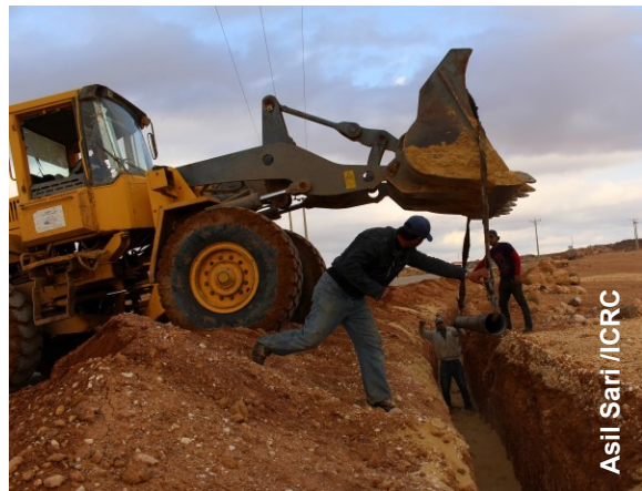
Work in progress on the rehabilitation of water transmission lines in North Badia.
