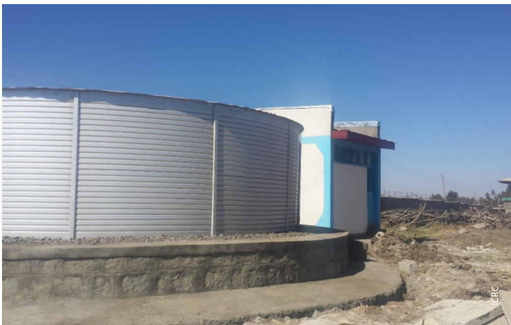
A 110 cubic-meter water reservoir and pump house built for Debre Birhan new prison, 2014.
