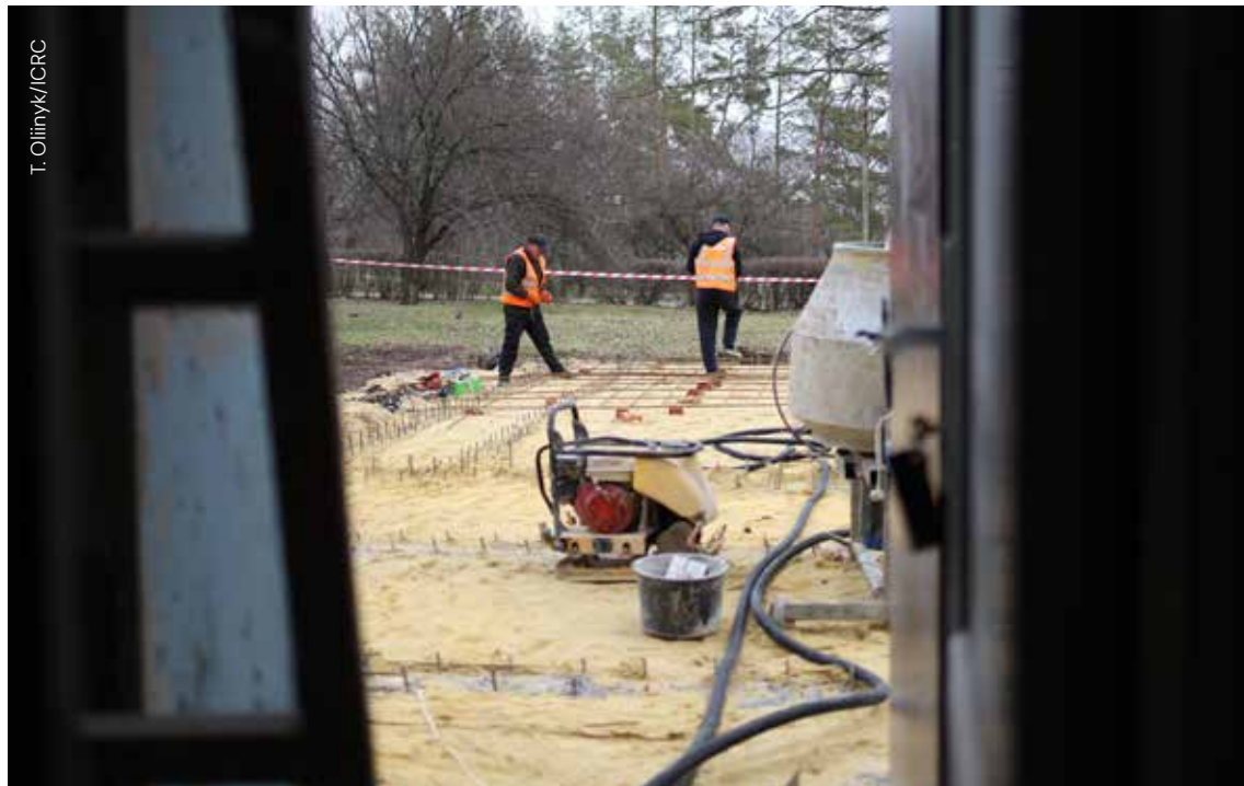
Central City Hospital, Kharkiv Oblast, Ukraine, March 2026. The ICRC is helping restore buildings at the hospital, to enhance conditions for patients and staff and improve infection control. This is particularly important, as the hospital receives large numbers of casualties, and conditions have a direct impact on their recovery.
