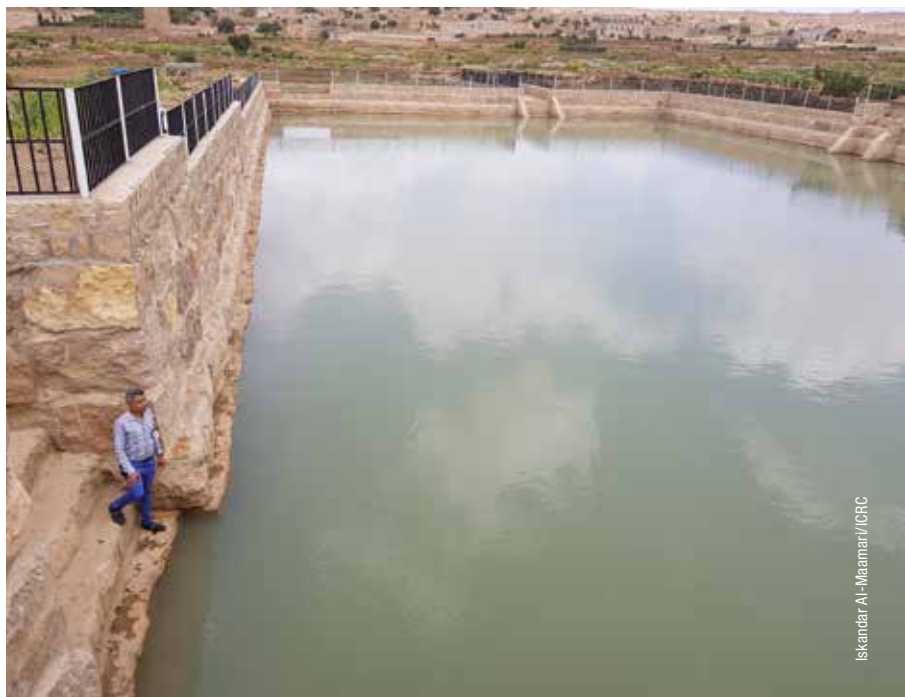
ICRC continues the rehabilitation of a water harvesting pond, started in 2018, in Arsham village in Arhab district north of Sana'a.
