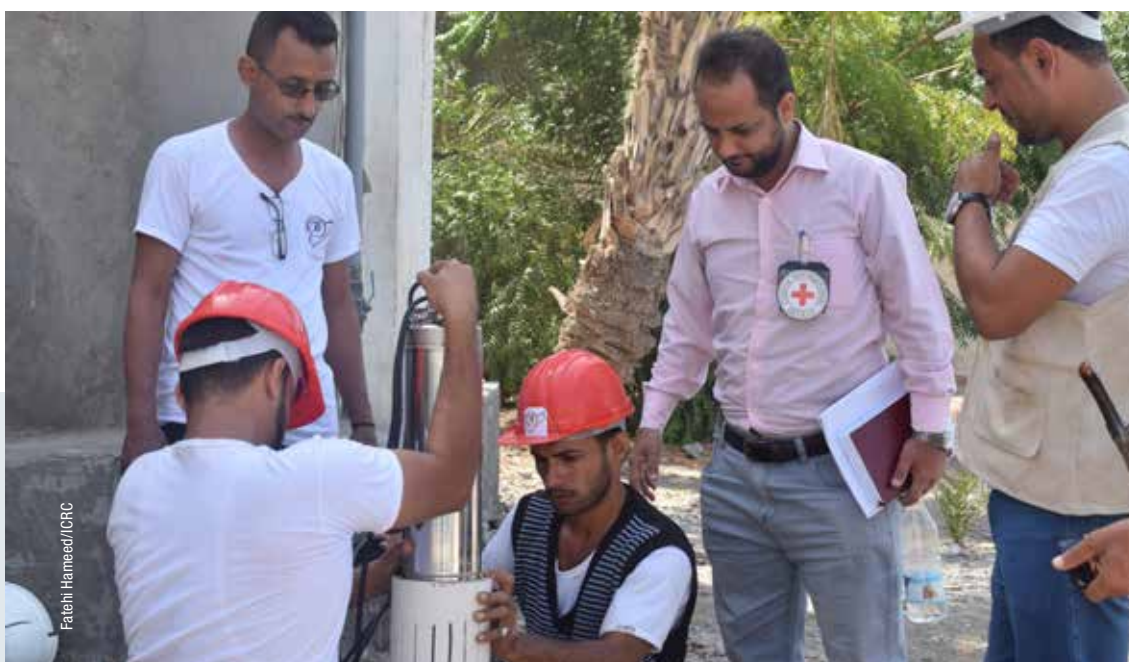
ICRC engineers install a submersible water pump which serves the emergency water-points project in Hodeida governorate.
