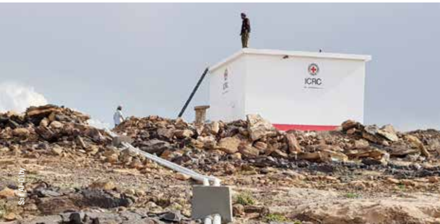
The reservoir of SAD Wathab Water Project in Akwan area of Al-Safra district in the governorate of Saada.
