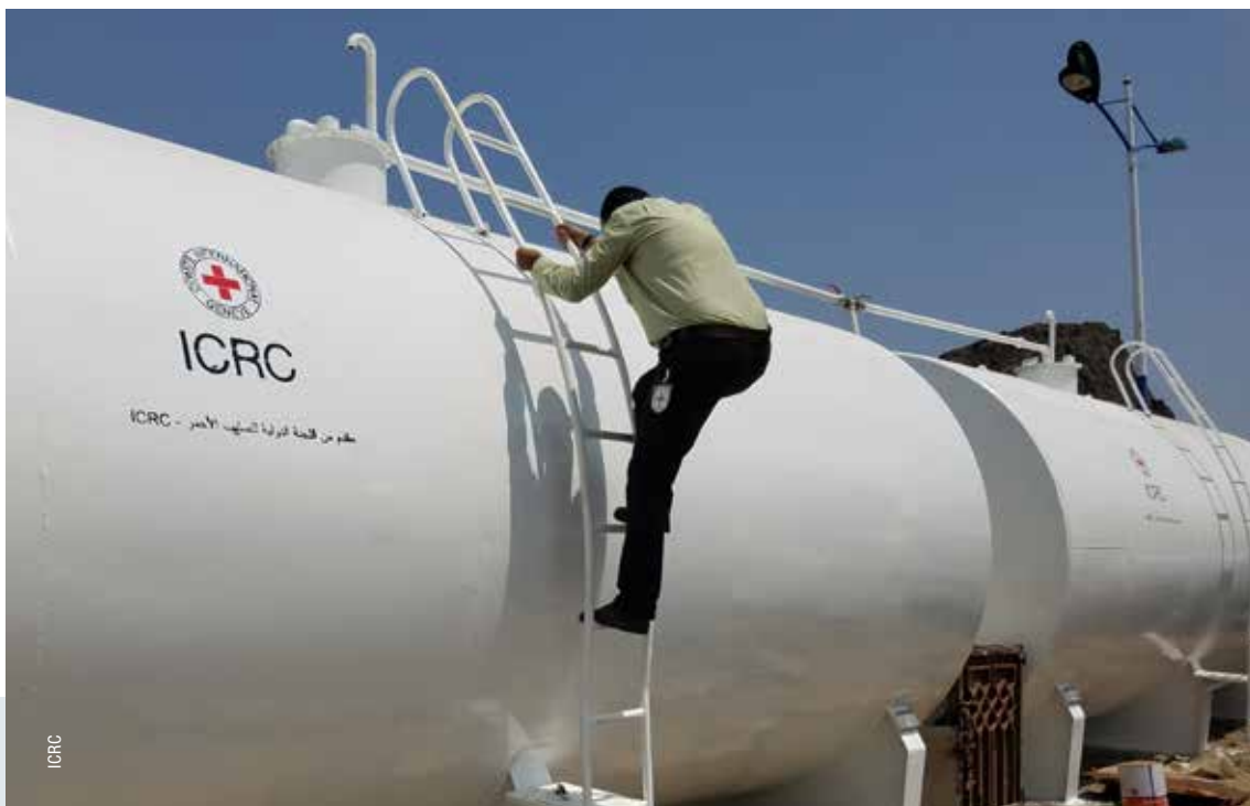
Two above-ground diesel tanks with the capacity of 50.000 liters donated to the Local Water and Sanitation Corporation in Taiz as a part of the ICRC constant support to the Corporation
