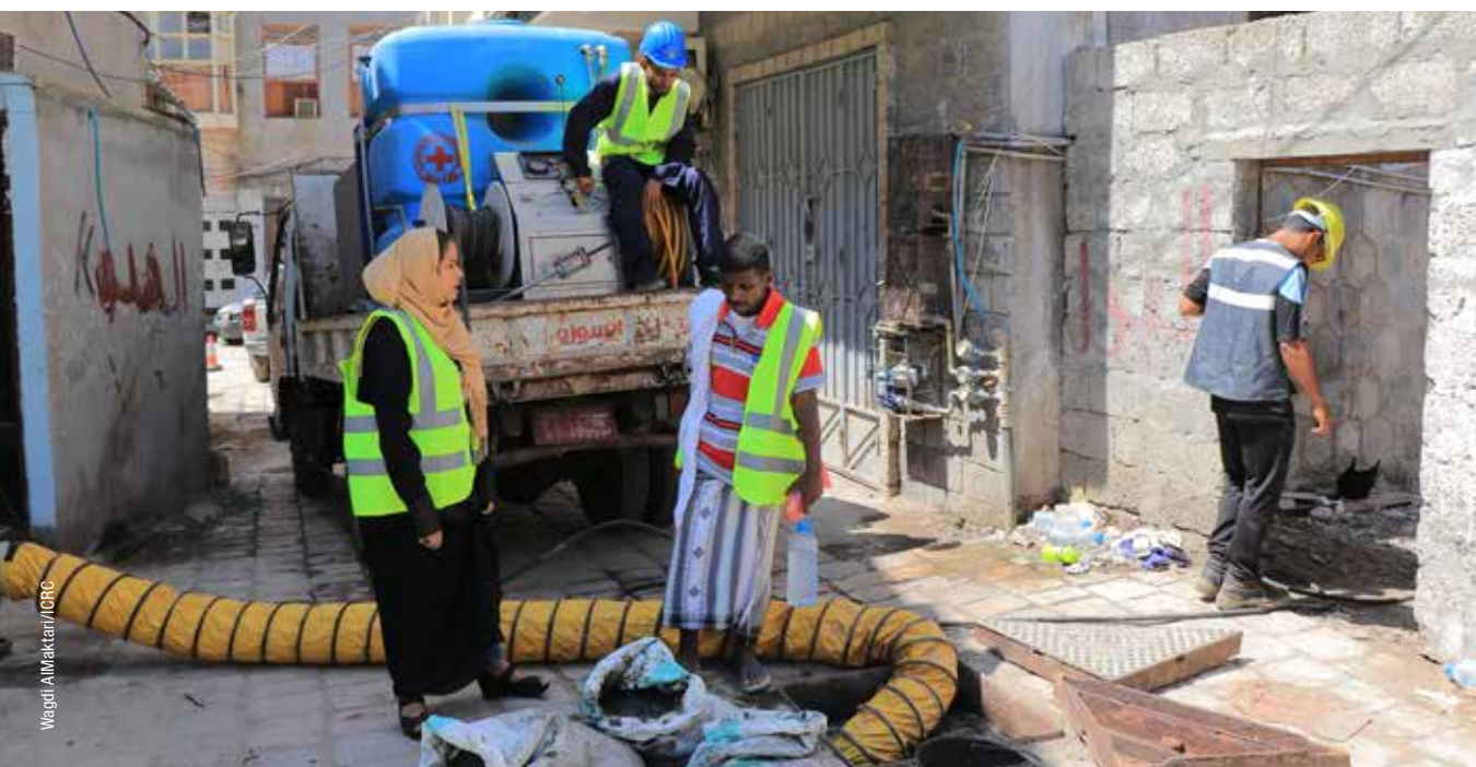
ICRC support Aden Local Water and Sanitation Corporation in with a jetting machine to remove sewage blockages
