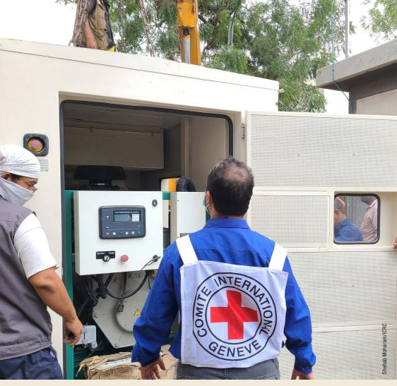
An ICRC engineer oversees the installation of a 130 KVA generator that the ICRC donated to the Local Water and Sanitation Corporation in Hodeidah as part of its regular support to the corporation.
